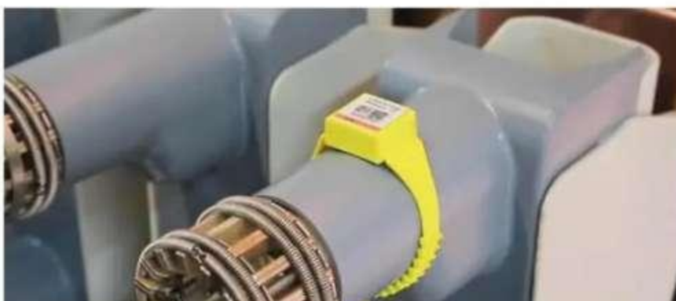
● Installed on Arm of Moving Contact
