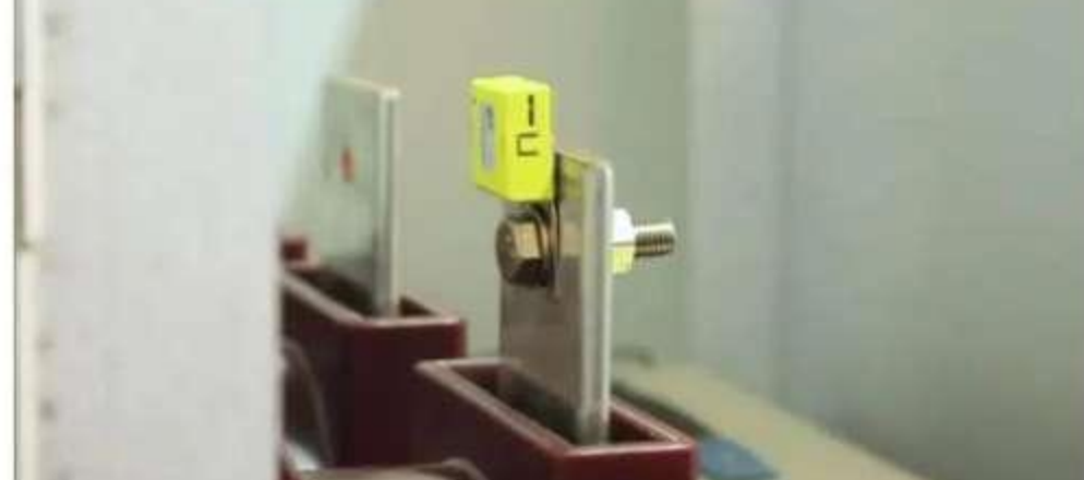
● Installed on Copper Busbar of Switchgear
