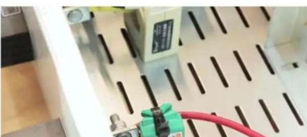
● Installed on Cable Joint of GCK Drawer
