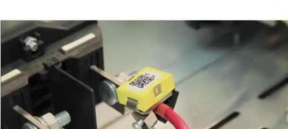
● Installed on Cable Joint of GCK Drawer
