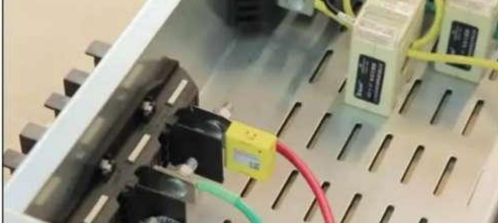
● Installed on Cable Joint of GCK Drawer
