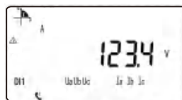
Voltage on A phase
